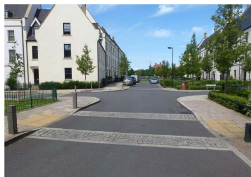
Figure 6.14: Street Precedents - Banding and flush conservation kerbs create a traffic calmed environment.
