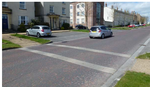
Figure 6.34: Banding and flush conservation kerbs create a traffic calmed environment
