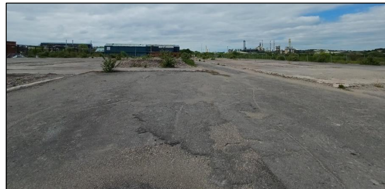
Barry Power Station (May 2025)
