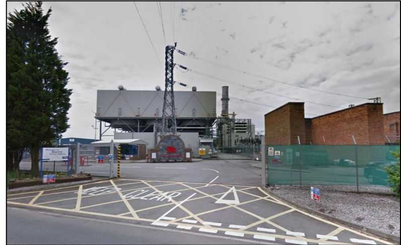
Previous Elevations of Barry Power Station
