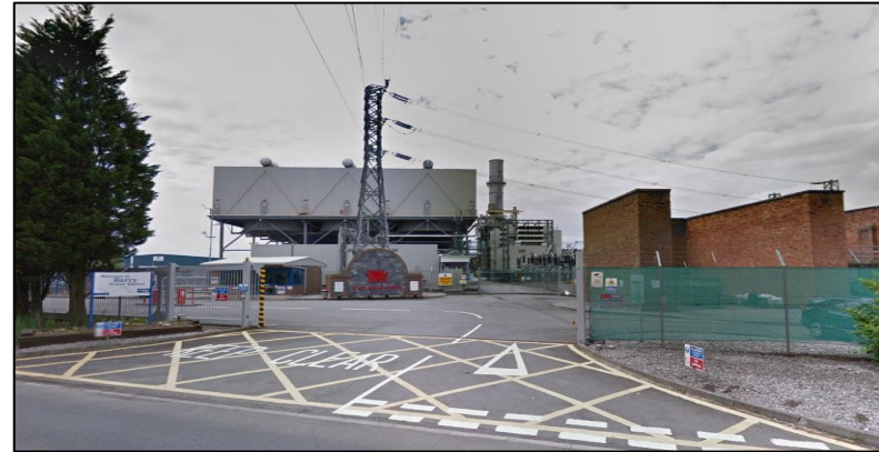
Barry Power Station (July 2012)
