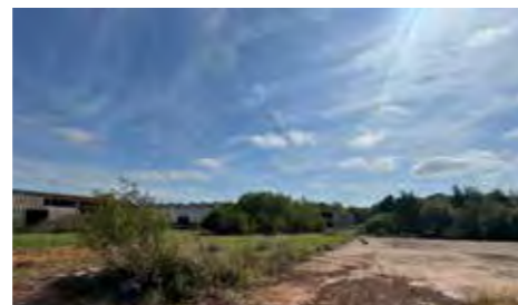
8 - View toward derelict buildings
