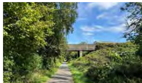
7 - Existing site access bridge over cycle route
