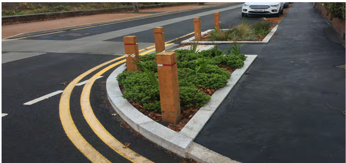
Figure 5 – Typical Bioretention System/ Rain Garden
