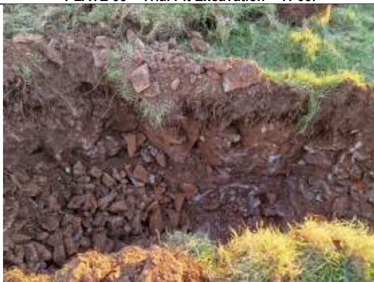
PLATE 07 – Trial Pit Excavation – TP04.
