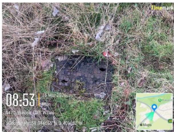
Photo 7: A view of drain cover along the north-eastern boundary.
