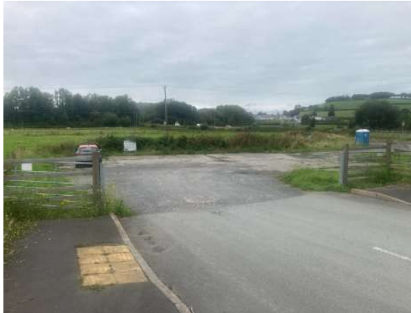
Photo 1: The southern boundary marked by the fencing, view showing the existing car park on site.
