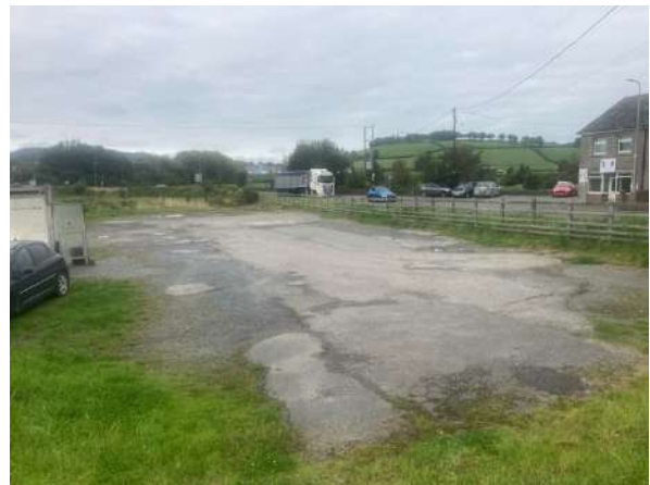
Photo 6: A view northward depicting the fencing which marks the eastern boundary of the site. The car park shown in the photograph is situated within the southeastern corner of the study area.
