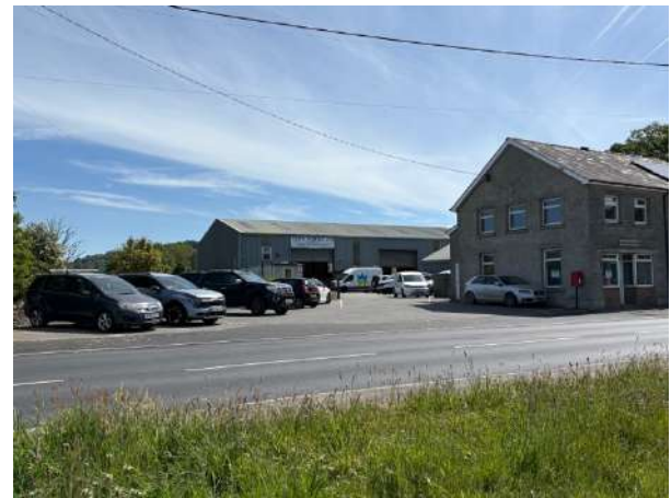
Photo 10: View eastwards from the eastern side boundary, towards the existing garage and site of the former tannery.
