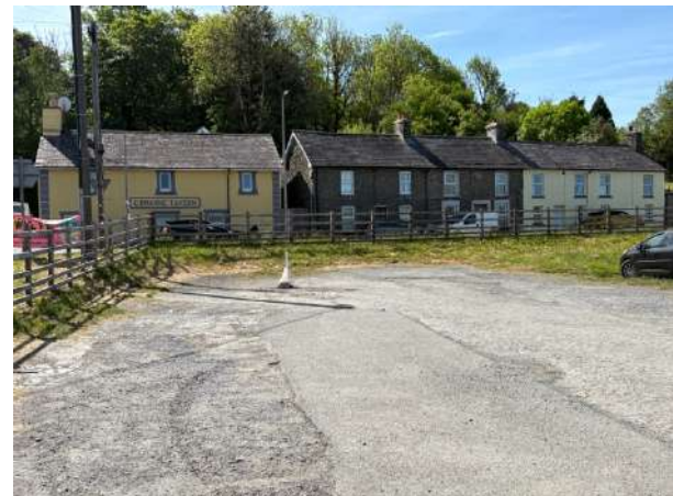
Photo 12: View southwards across the existing car park area.
