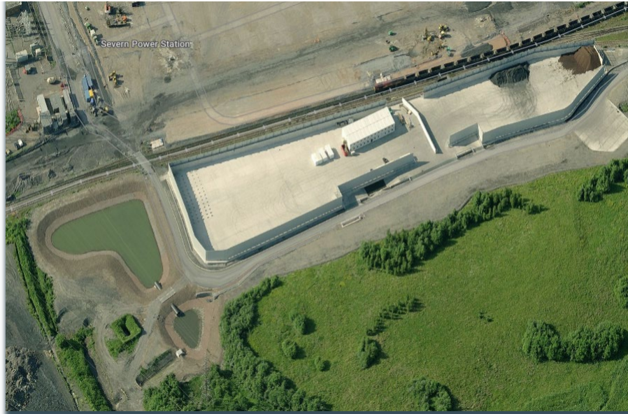
Figure 3: Aerial Image of PFA Storage Area
