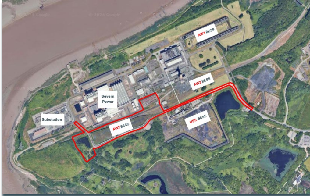
Figure 2: Aerial Image of Proposed BESS Site
