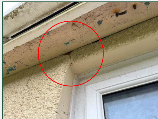
IMAGE 8: GAP UNDER SOFFIT
